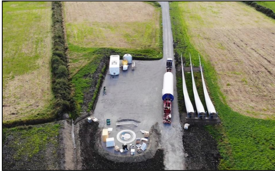
Plate 4-9: Typical finished hardstand on a wind farm
