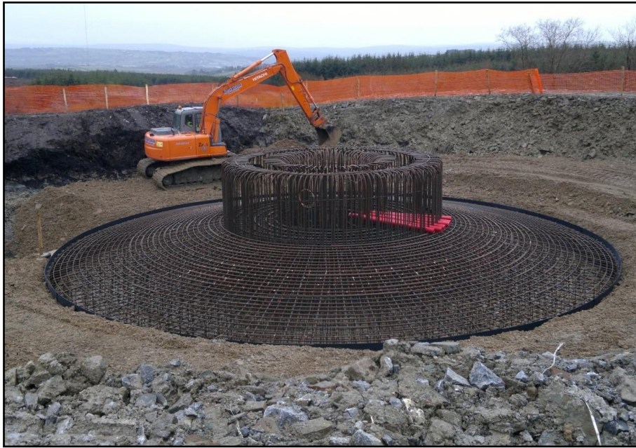
Plate 4-10: Typical construction of a wind turbine base
