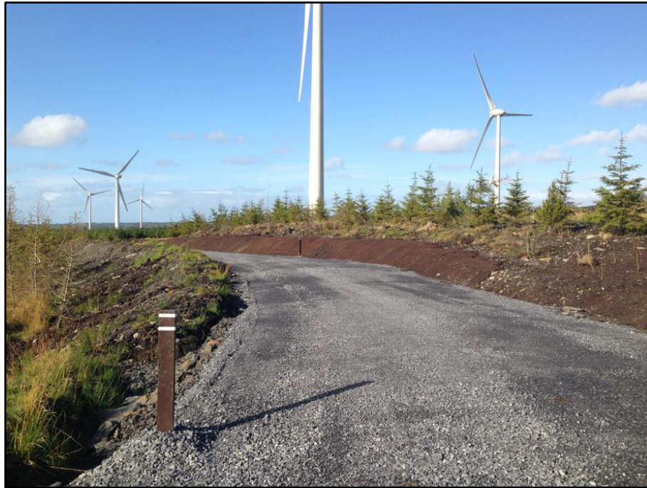
Plate 4-2: Typical new excavated access track on a wind farm
