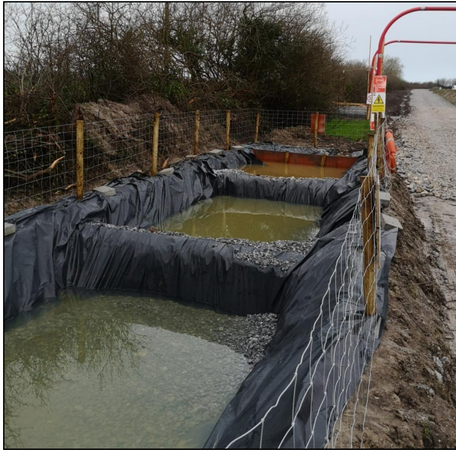
Plate 4-7: Construction stage wind farm sediment settlement pond
