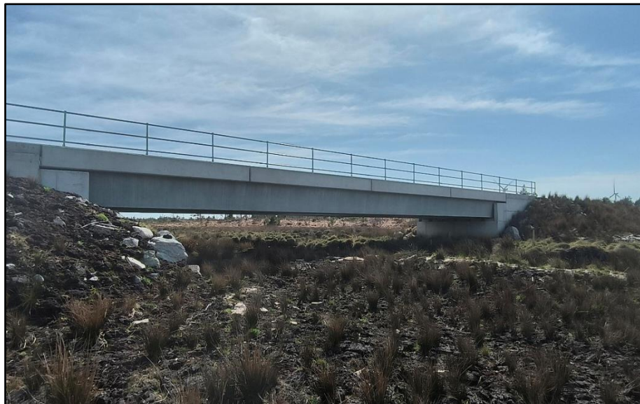
Plate 4-8: Completed Clear-Span Bridge over existing watercourse
