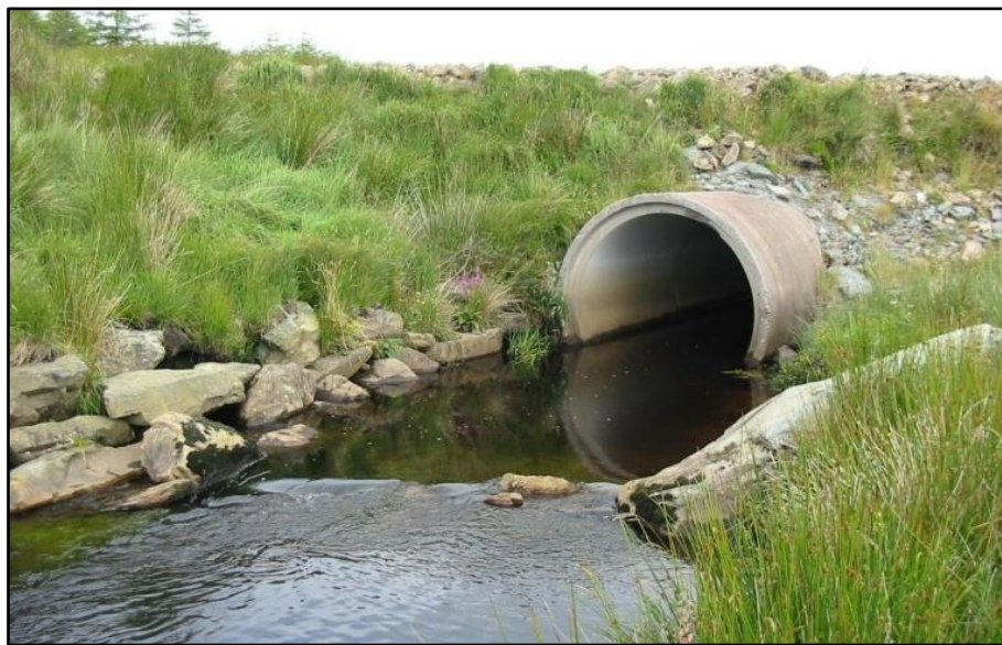
Plate 4-4: Typical surface water drain crossing
