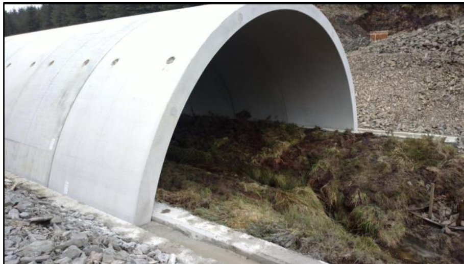
Plate 4-5: Typical clear span pre-cast concrete units in place over an existing watercourse
