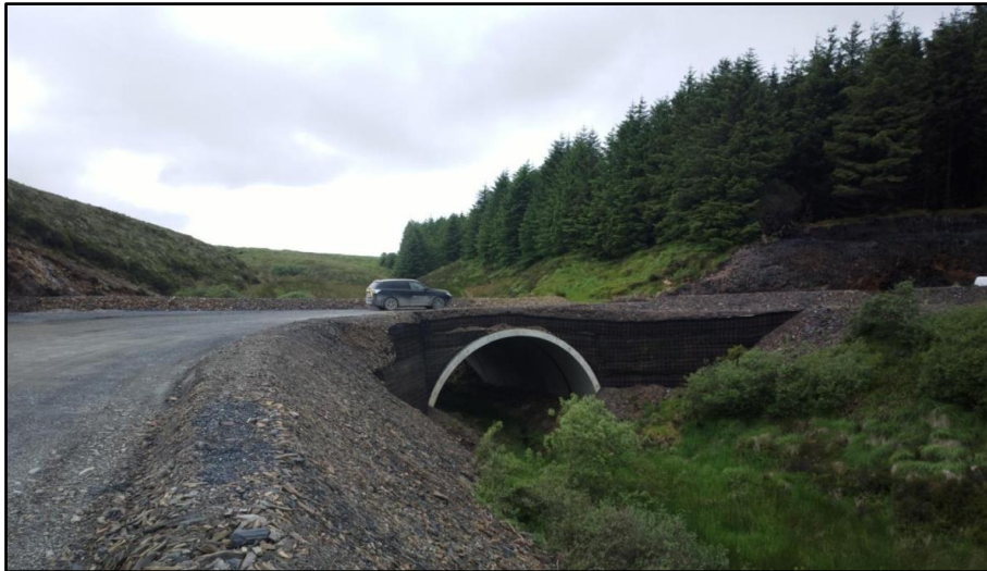
Plate 4-6: Completed clear span pre-cast concrete culvert over existing watercourse
