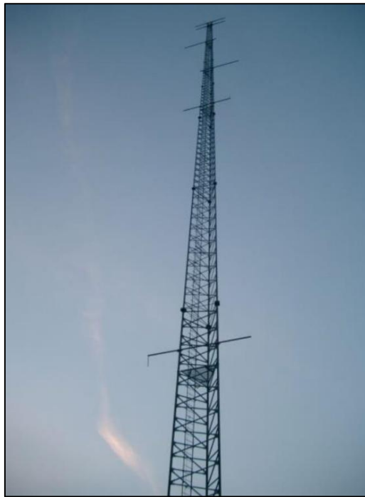
Plate 4-12: Typical meteorological mast on a wind farm
