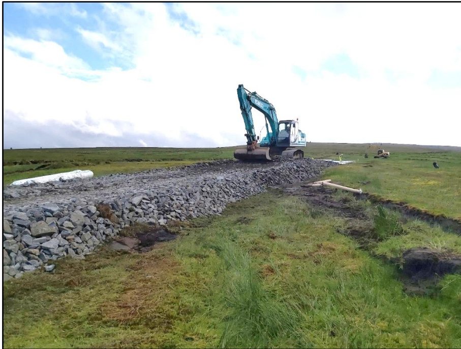
Plate 4-3: Typical floated track on a wind farm
